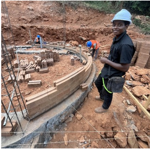
Paul Ikocha building a small guest house using the same type of compressed bricks he will use on the School of Nursing project
