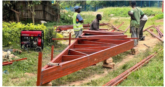
Trusses are now ready to be mounted.
