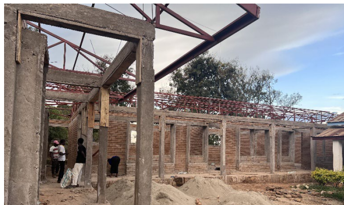
The roofing structure and roofing are now being installed. The final phase will be the installation of doors, windows, and finishing of the walls.
